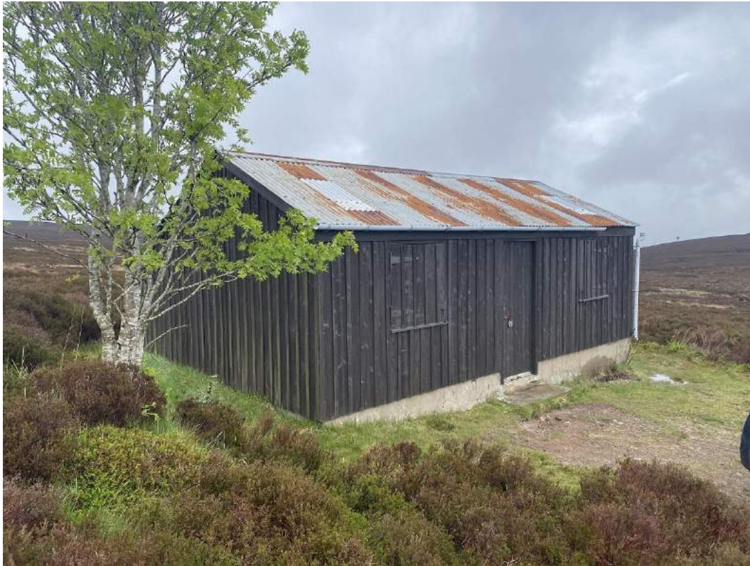
Plate 3: Modern bothy located on existing track (TN5)
