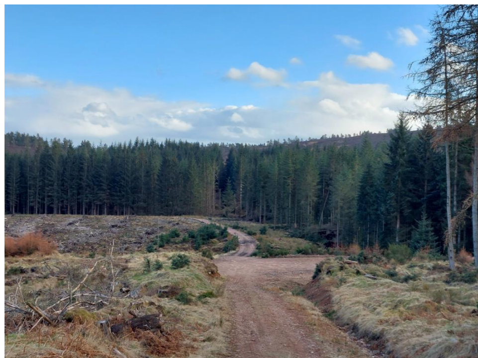
Photograph 3: View south towards Control Building & Substation and BESS.
