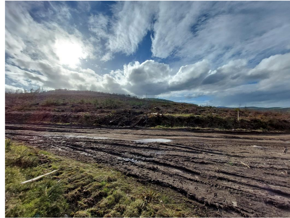
Photograph 1: Temporary Batching Plant Location looking west towards Hill of Fare.
